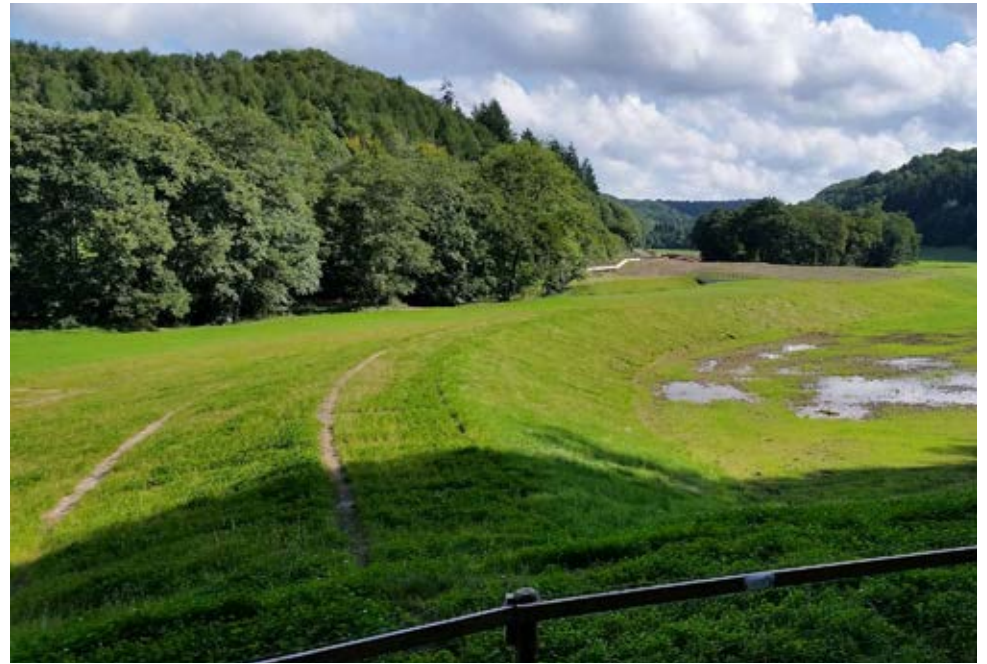
Top: View of completed low-level berm following revegetation of grasscrete surface. (Photo by Tom Nisbet, Forest Research)
