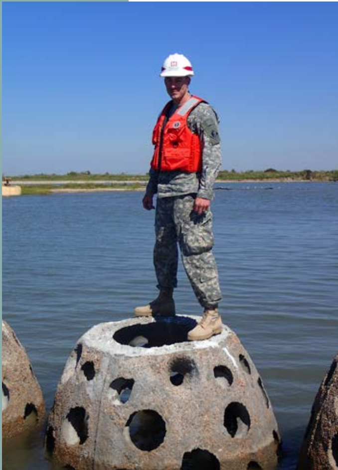
Left: Goliath Reef Balls were installed to protect natural shorelines and provide habitat near the Gulf Intracoastal Waterway in West Galveston. (Photo by ERDC)
