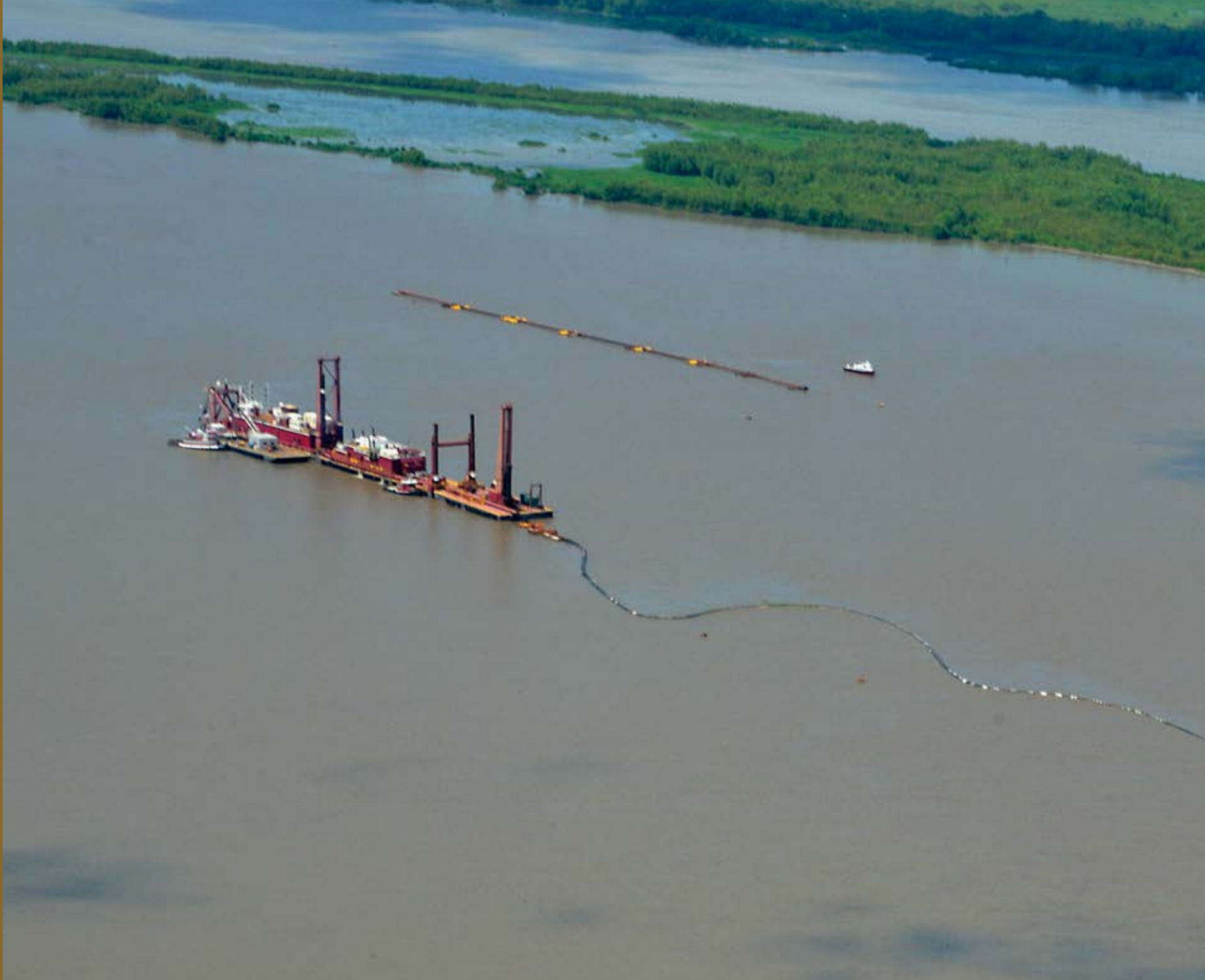
Behind the dredge California, the river island at Horseshoe Bend on the lower Atchafalaya River, Louisiana, is being self-designed by the strategic placement of sediment upriver (lower right), which allows the river's energy to disperse the sediment. The dispersed sediment contributes to the island's growth, thus creating environmental and other benefits. (Photo by Wings of Anglers, courtesy of Great Lakes Dredge and Dock Company)
