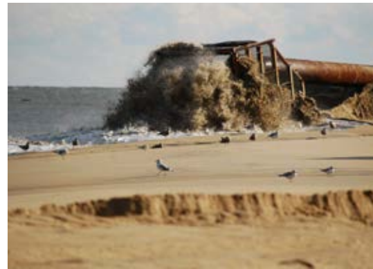
Below: The USACE Philadelphia District is renourishing Dewey, Rehoboth, and Bethany Beaches, Delaware, as part of a regular project in 2011–2012. Work was completed at South Bethany Beach, Fenwick Island, and Lewes, Delaware, in 2011. The projects are designed to reduce storm damage to public and private infrastructure. (Photo by Ann Cameron Siegal, USACE Philadelphia District)
