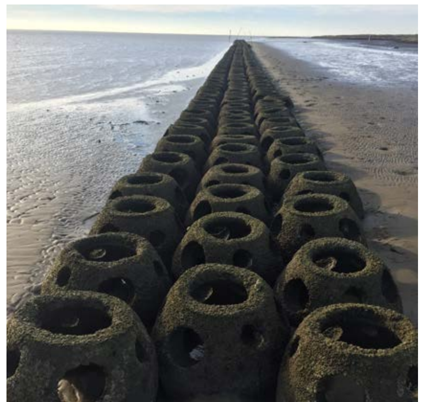
Top: Oyster reef breakwater constructed from ReefBLK. (Photo by Mary Kate Brown, The Nature Conservancy)
