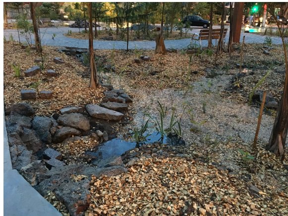
Figure 68. After the planting, storm water of 1 000 m 2 of paved surface was conducted to the rain garden and infiltrated, avoiding recurrent floods in the region.
