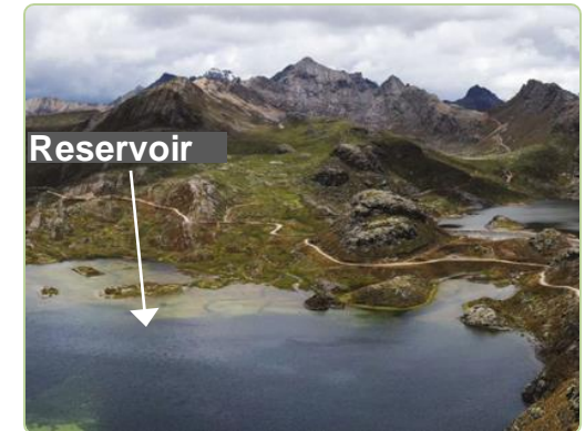
Water reservoir constructed for water security in the Andes
