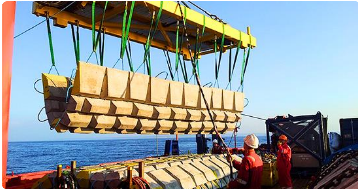
Roman Stone Construction Co. marine mattress being installed in the United Kingdom 75
