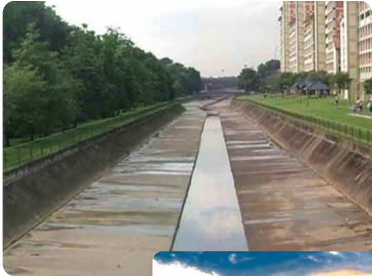
Original concrete- lined canal
