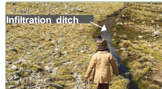
Ditches constructed for water infiltration
