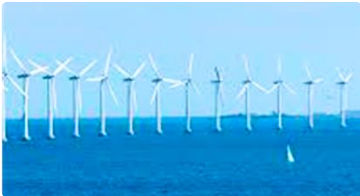
Wind turbines installed with use of EConcrete 67
