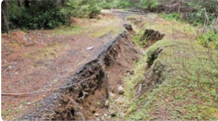
Removal of culverts on an unused road
