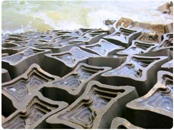
EConcrete used in a coastal fortification structure 66
