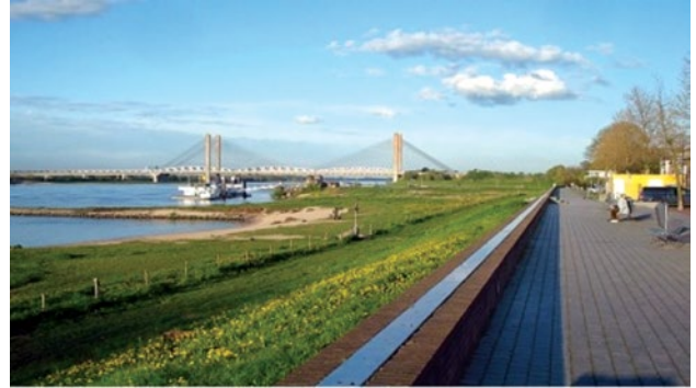
Horizontal levee to protect from riverine flooding in Zaltbommel, Netherlands (flood wall on the dyke Voorendt, 2015 ).
