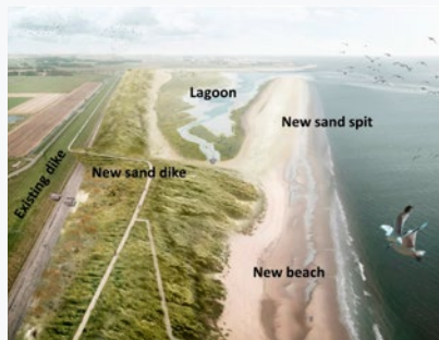
Artist impression new Prins Hendrik sand dyke (Source: Feddes and Olthof in litt. Perk et al. 2019 143 )
